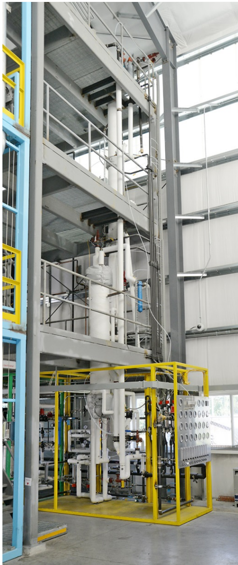
RTI's Bench-scale Prototype System in USA
